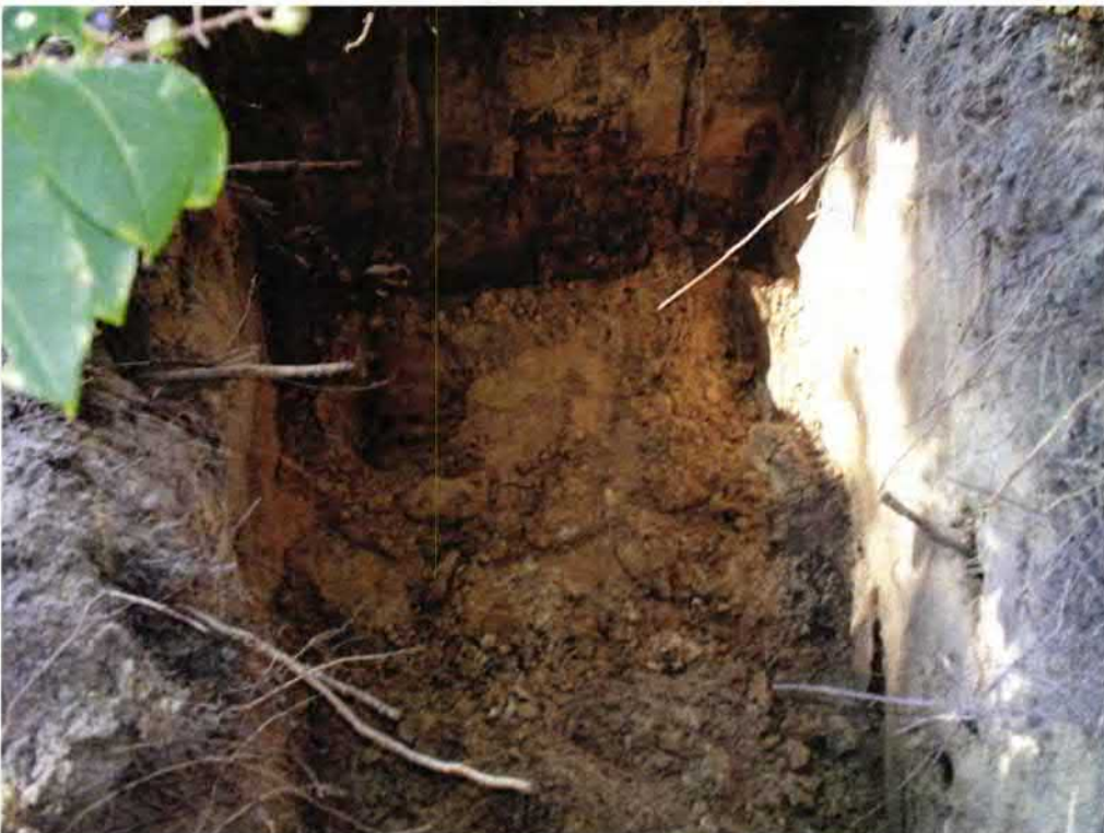
Picture 2: UST 822Azalea excavation.
